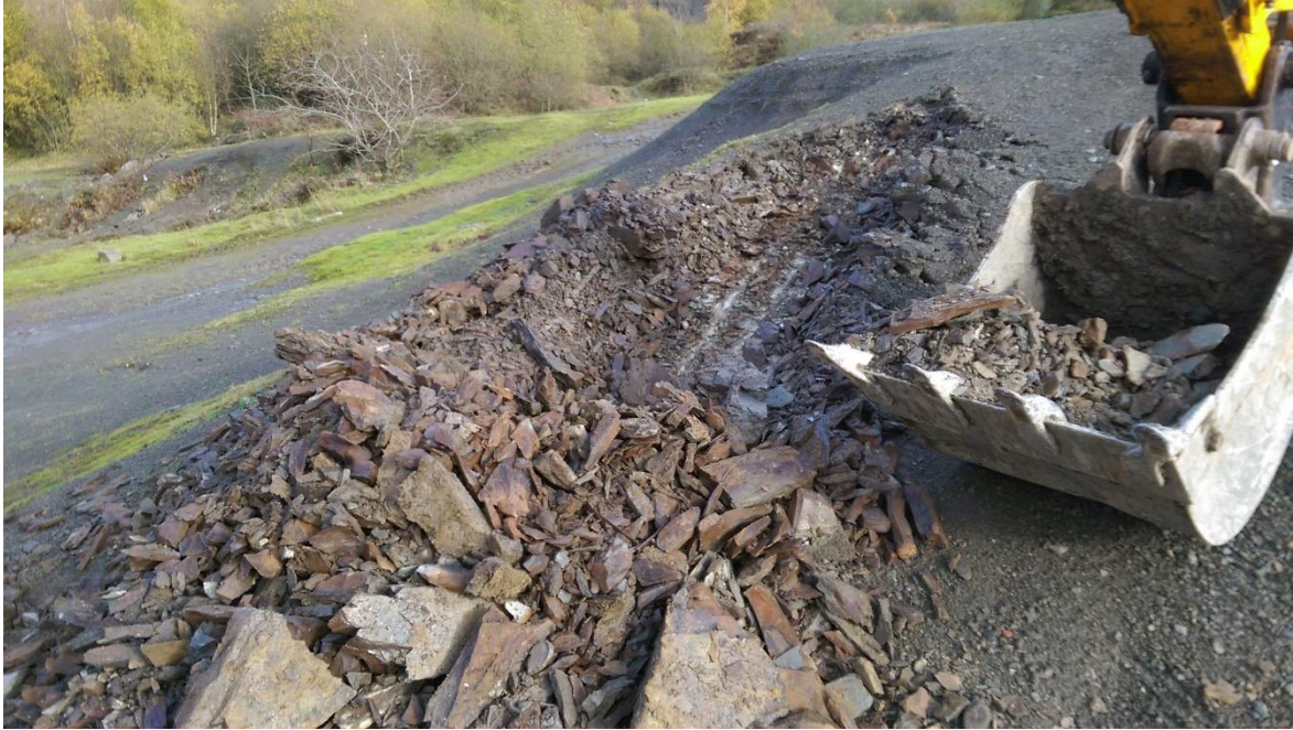
Photo 3: Mudstone bedrock encountered directly beneath the surface in the quarry floor.
